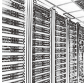
Server power supply
